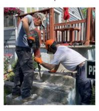
Many thanks to all who helped remove the existing concrete stairs to the caretakers' quarters. This was a very labor-intensive project that saw 4 metric tons of concrete broken up and removed. The new stairs are to be installed in early July.
